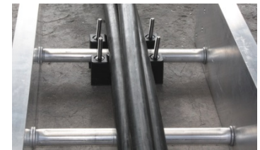
Figure 2 Cable Cleat Base Below Rung
